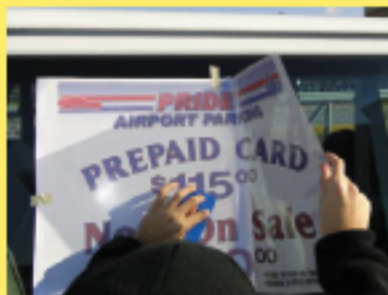
STEP 6. Gently apply perforated material with squeegee, always squeegee from center to outer edges.
