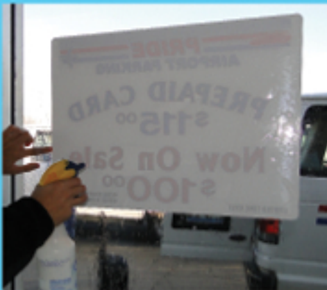
STEP 6. Keep spraying the graphic. Slide graphic around until it is where you want it.
