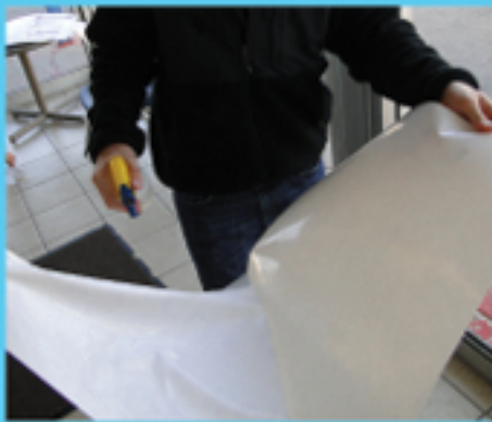
STEP 3. Keep applying water as you take the liner completely off.
