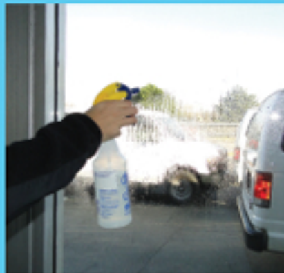
STEP 4. Clean glass thoroughly and wet glass completely over application area.
